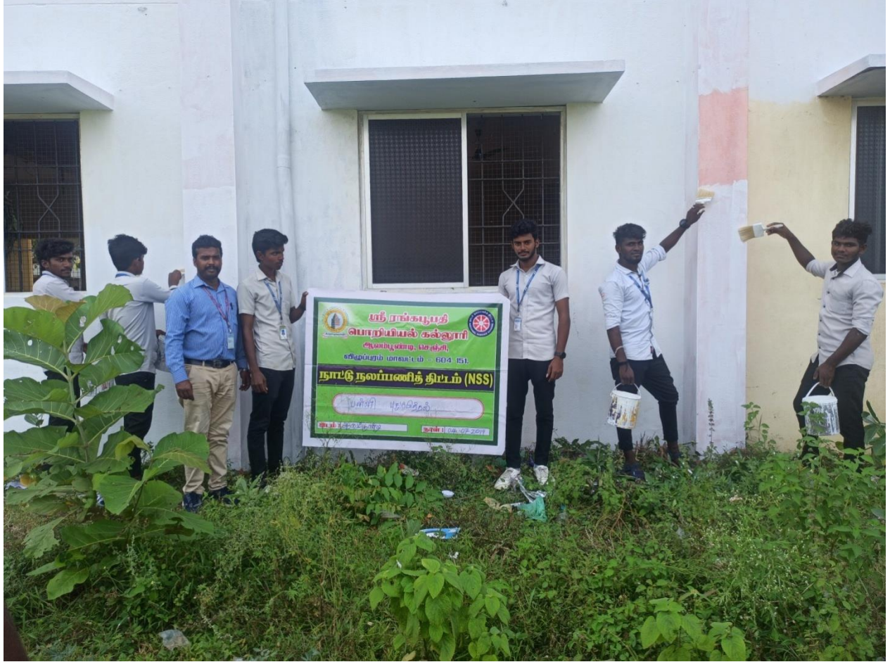
GOVERNMENT SCHOOL RENOVATION PROGRAM AT ALAMPOONDI VILLAGE ON 02.09.2019
